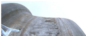
Slight hollow wear and some fatigue cracking from KTH Royal Institute of Technology www.kth.se
