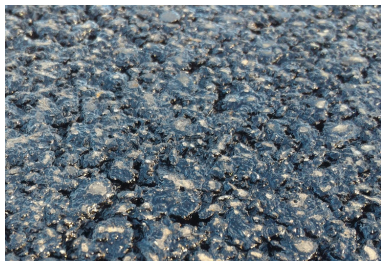
Very fresh asphalt concrete
