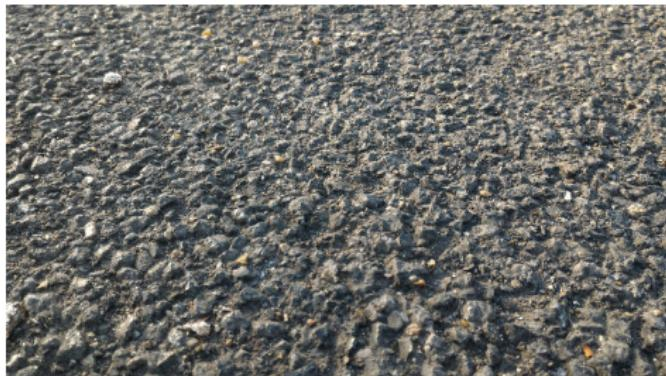
Old asphalt concrete with worn out bitumen
